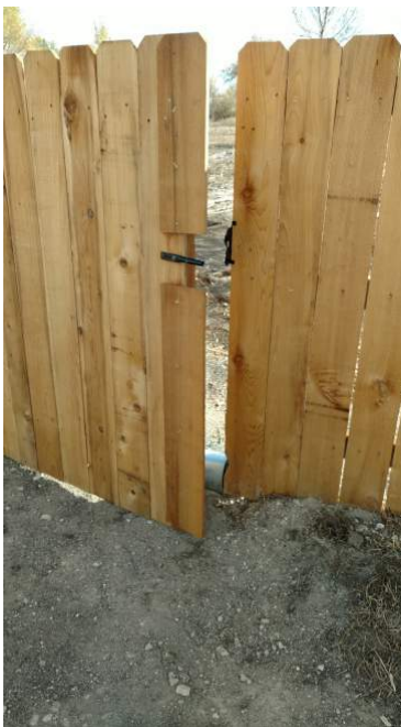
Overlay board at edge of gate so when closed there is no light penetration.
